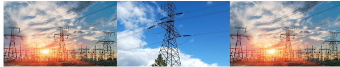
Long span fiber optic cable
